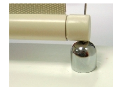
13mm gap under round hem bar
