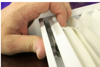
21 Whilst under tension, place headrail over the brackets.
