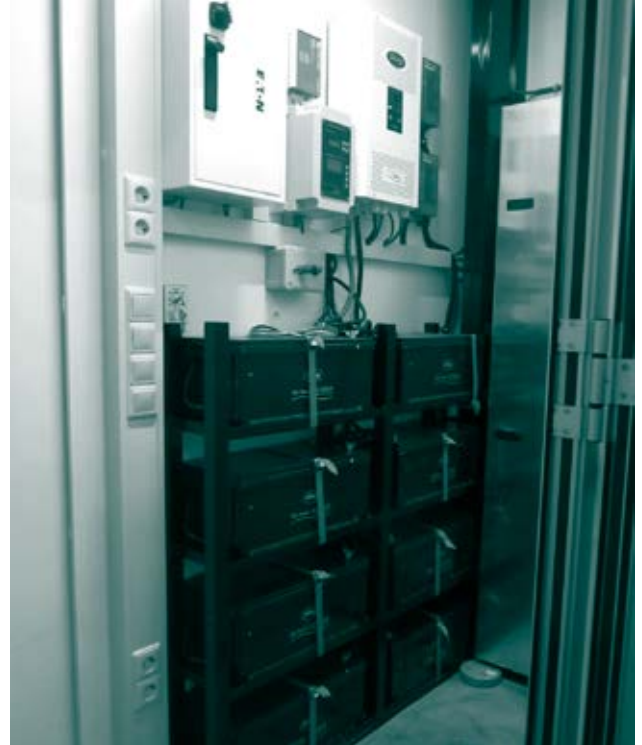
Typical example of an AGM battery bank powering a 3.5 kW inverter
